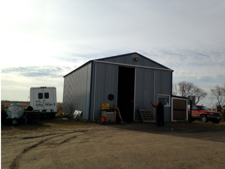
Photo 11: Depot at Newdale Landfill
